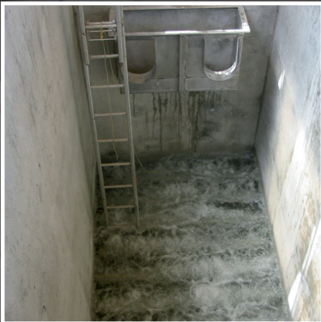
Warkworth WTP - mechanical plant Fabricate, supply and install Rodney District Council
